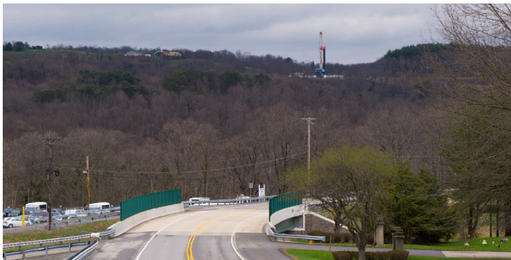
Exhibit 10.2 Building an overpass or road bridge is a complex and multidimensional process involving equipment and materials from dozens of entities. Earth movers, cranes, drainage and sewers, safety components, gravel, cement, and large objects such as steel girders must all be transported to the site according to a tight schedule and specific budget. And then the workers, engineers, and inspectors must be sourced, scheduled, and compensated. This work is done at multiple locations, all at once, in every state in the country. Operations managers are core to making it happen. What are the key inputs in the road construction process? (Credit: Mark Dixon/ Flickr/ Attribution 2.0 Generic (CC BY 2.0))
